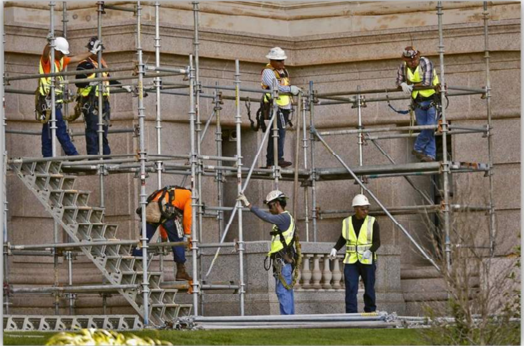
Trial Area Scaffold Erection
