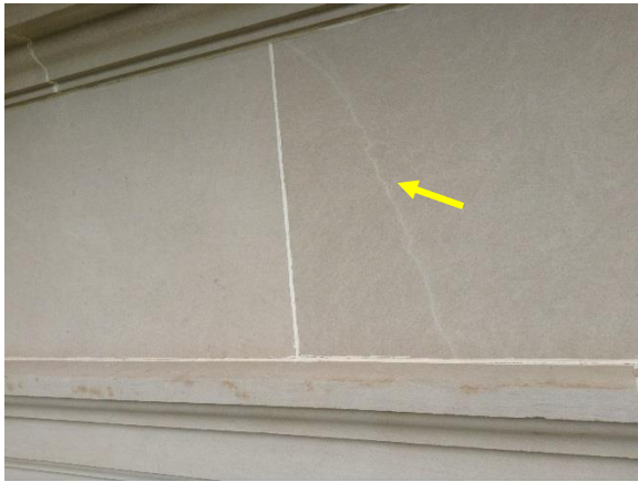
Figure 33. Seam within limestone unit
