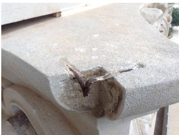
Figure 31. Area of limestone dutchman repair removed during inspection
