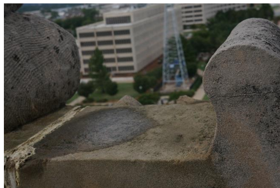
Figure 73. Area of trial cleaning at limestone parapet after application of cleaner
