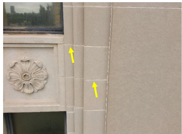
Figure 26. Mortar bond failure between limestone units
