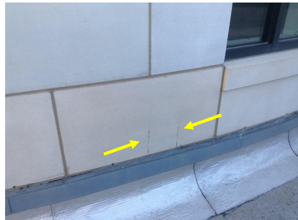
Figure 132. Parallel cracks within dome base cast stone unit
