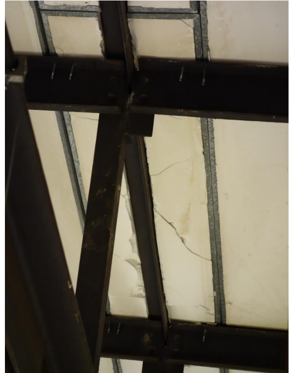
Figure 106. The gypsum panels above the House chamber are cracked.
