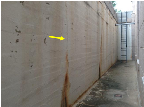
Figure 42. Cracks at foundation walls
