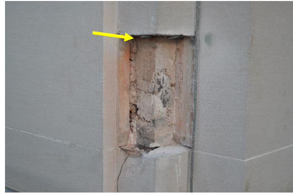
Figure A34. Anchor within jamb unit
