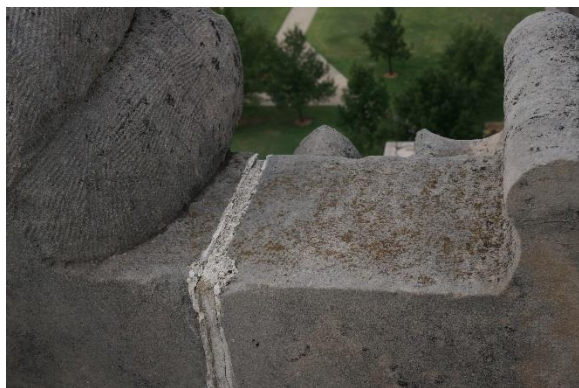
Figure 72. Area of trial cleaning at limestone parapet before application of cleaner
