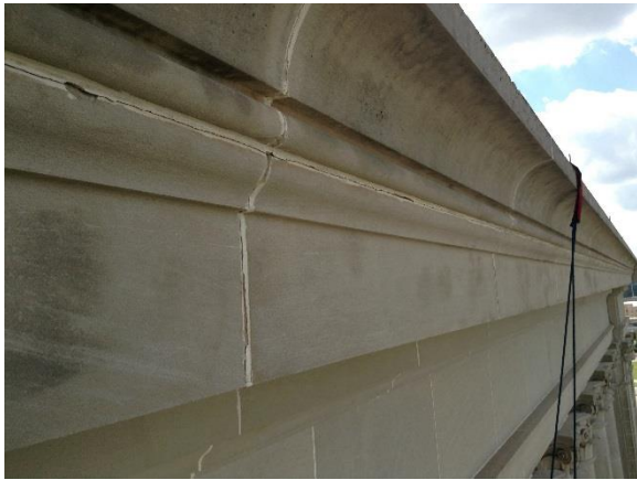
Figure 27. Cementitious coating at mortar joints
