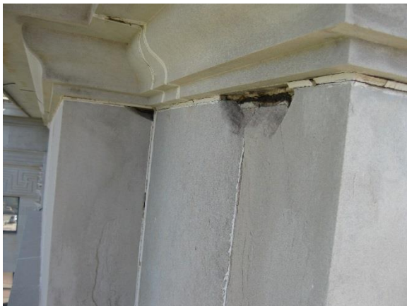
Figure 13. Example of limestone spall at frieze panel
