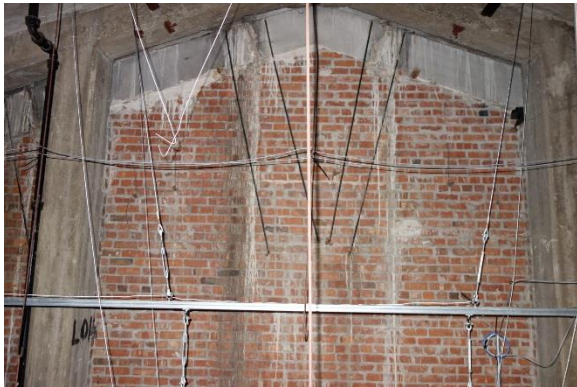
Figure 107. The metal straps that engage two levels of projecting stone work on the exterior of the north gable (above)
