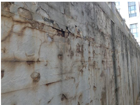
Figure 43. Cracks and spalls at foundation walls
