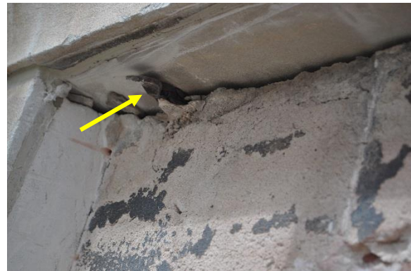
Figure A36. Strap anchor within opening
