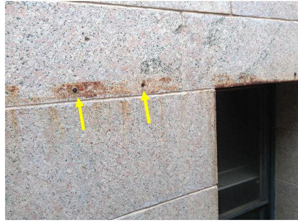
Figure 37. Close-up view of abandoned anchors
