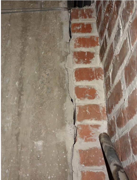
Figure 105. Crack between the brick wall and concrete frame at west gable
