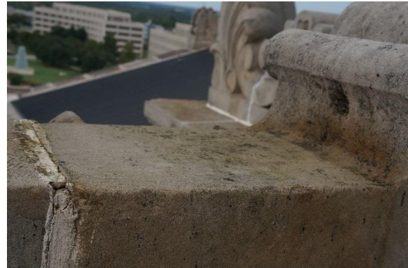
Figure 75. Area of trial cleaning at limestone parapet after application of cleaner
