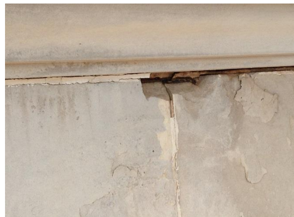
Figure 14. Close-up view of limestone spall coincident with original strap anchor
