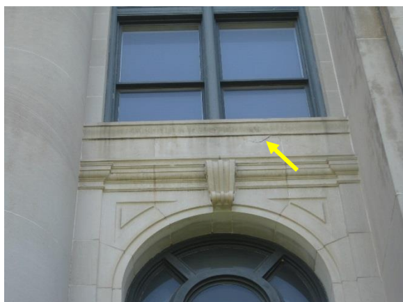
Figure 19. Example of limestone spall at spandrel panel
