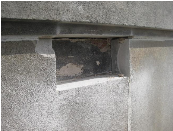
Figure A10. Lack of strap anchor within opening
