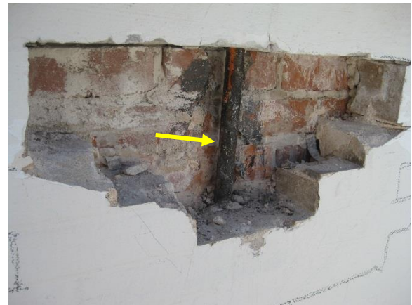
Figure A13. Minor corrosion on cornice rod
