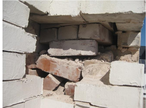
Figure A23. Loose masonry within pilaster
