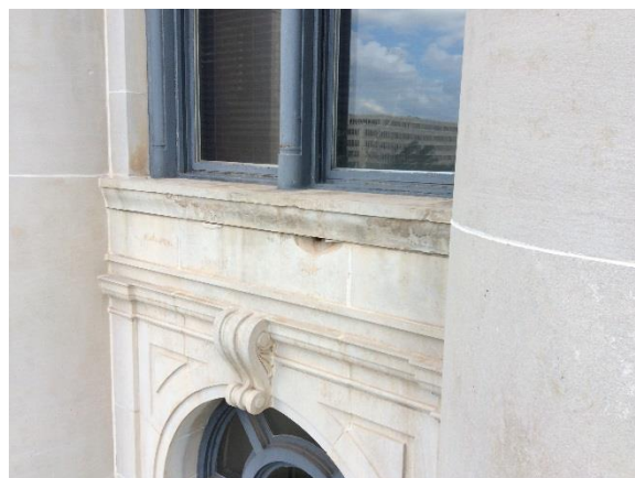
Figure 18. Example of limestone spall at spandrel panel
