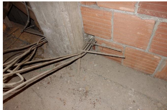
Figure 96. Typical tieback of the wire cables to the concrete frame
