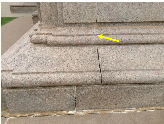
Figure 34. Crack within granite unit
