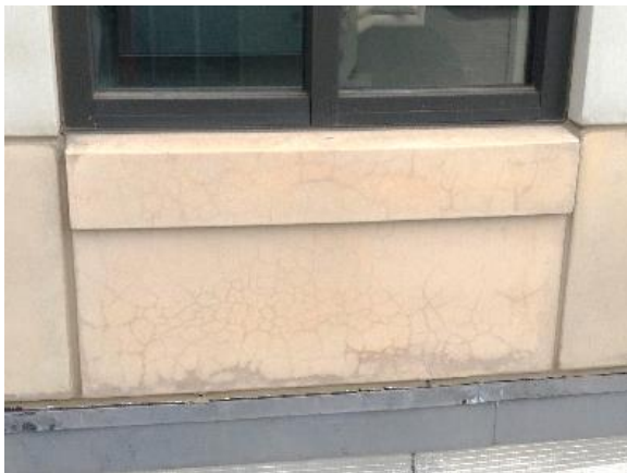
Figure 135. Craze cracking at face of cast stone unit at base of dome
