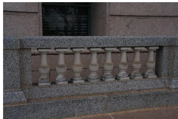
Figure 62. Stained limestone balusters
