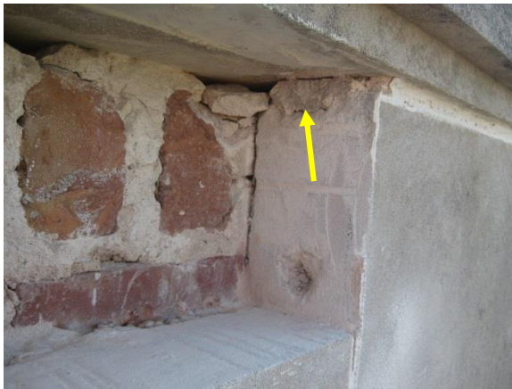
Figure A28. Lack of anchor within opening
