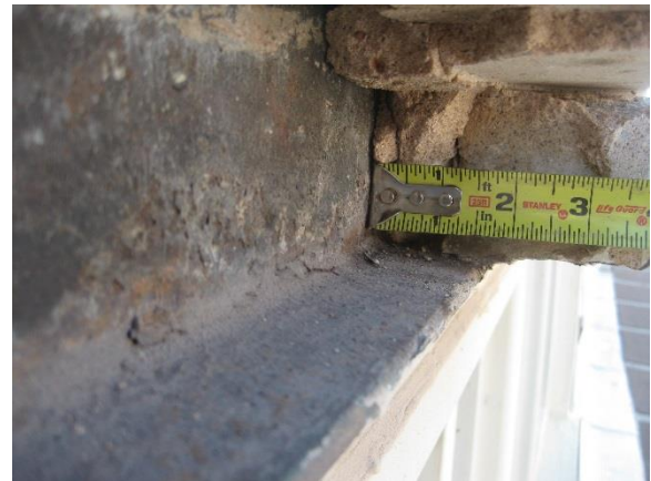
Figure A25. Bearing of brick on lintel
