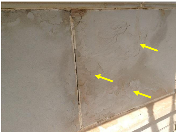
Figure 29. Exfoliation of limestone units
