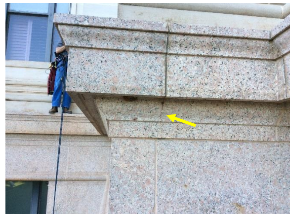
Figure 35. Crack within granite unit
