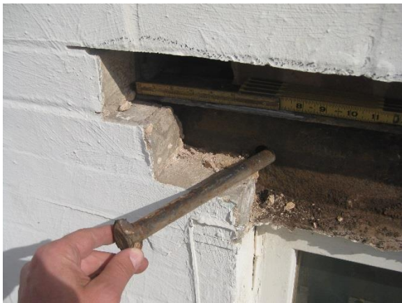
Figure A9. Unengaged bolt at lintel
