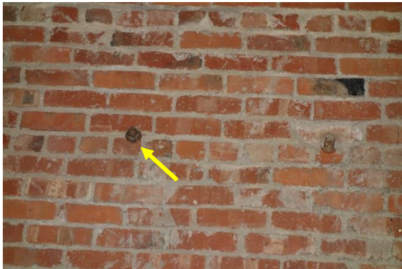
Figure 99. Through-bolt anchors present on the inside of the south gable wall
