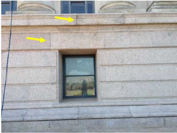
Figure 38. Washed-out mortar in granite units
