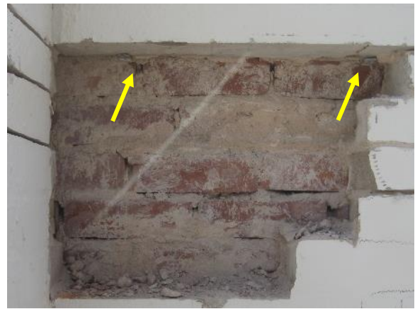
Figure A5. Galvanized ties within brick masonry
