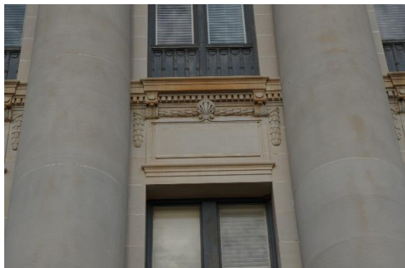
Figure 53. Dark orange staining of limestone at window sill (above)
