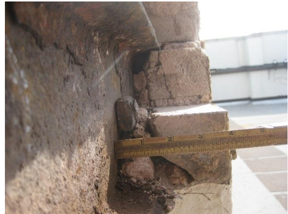
Figure A8. Bearing of brick on lintel below
