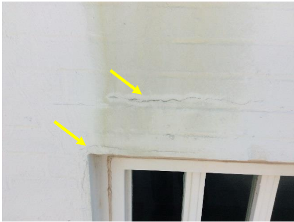
Figure 84. Close-up view of spalling and cracking of brick above clerestory windows
