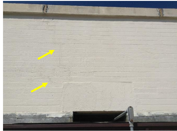
Figure 85. Cracking at back face of masonry walls
