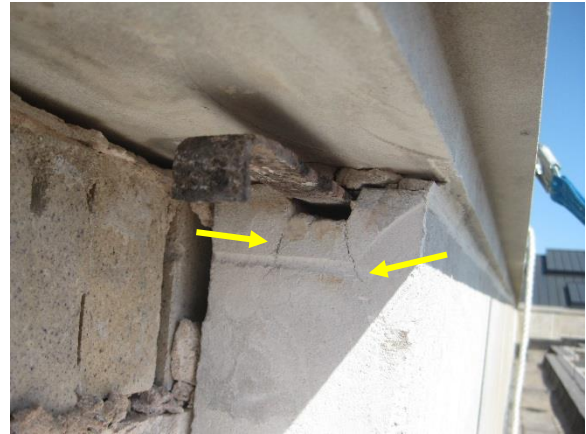
Figure A18. Cracking at kerf within unit
