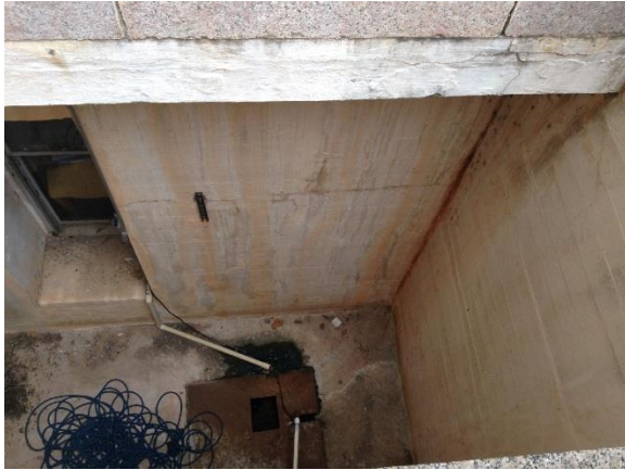
Figure 40. Coating applied to light well walls
