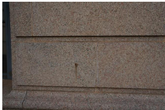
Figure 64. Staining from ferrous mineral inclusions
