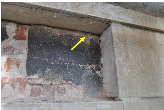
Figure A37. Lack of strap anchor within opening
