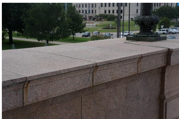
Figure 65. Staining of granite from surface-applied metal appurtenances
