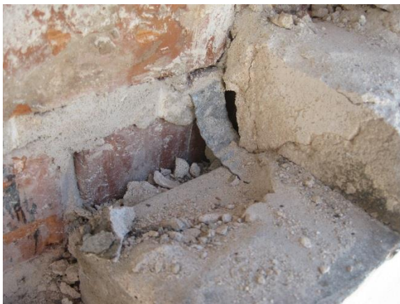
Figure A14. Typical corrugated masonry tie
