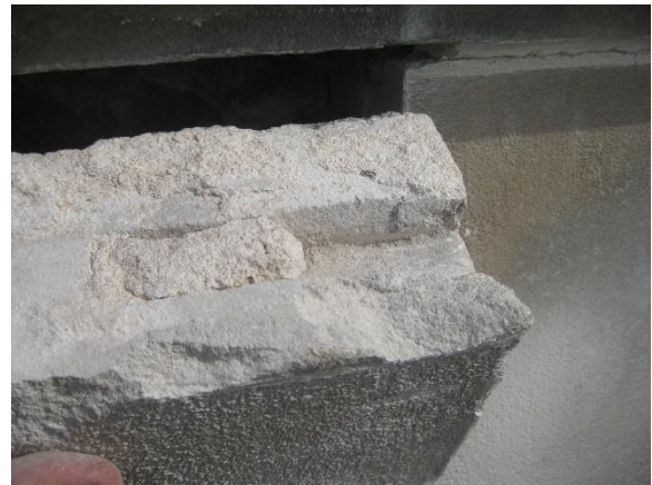
Figure A11. Lack of strap anchor within opening
