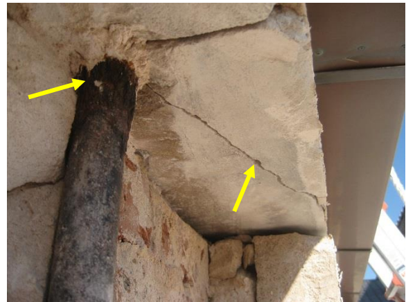
Figure A21. Corrosion scale on surface of cornice rod
