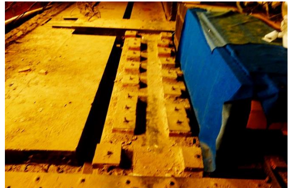
Figure 100. Heavy steel framing on the floor of the south attic between the concrete frame and masonry wall supporting the south portico soffit
