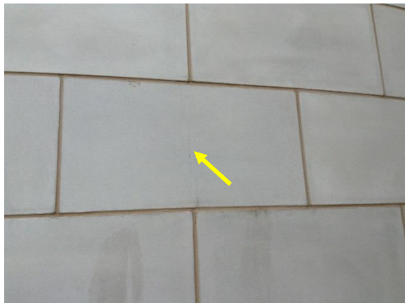
Figure 131. Crack at cast stone near center of dome base unit
