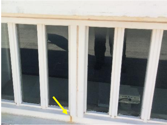
Figure 88. Corrosion staining at clerestory windowsill
