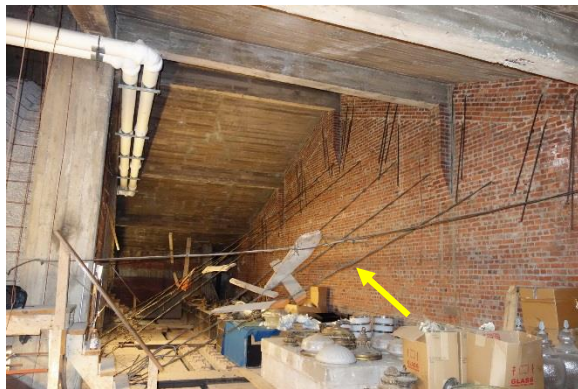
Figure 95. View of the back side of the south gable showing wire cable ties to concrete structure
