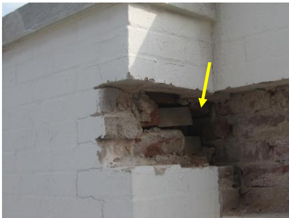
Figure A6. Lack of tie between pilaster and wall
