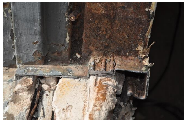
Figure 118. Section cut at the steel sill
