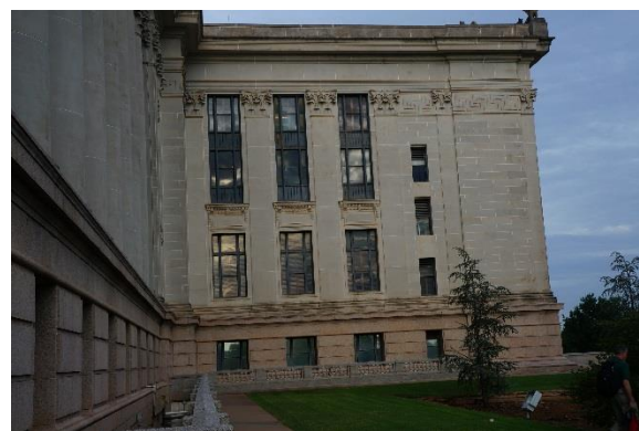
Figure 60. Dark staining at limestone parapets
