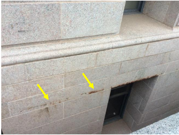
Figure 36. Corrosion staining at abandoned anchors at light wells
