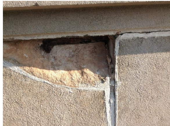
Figure 12. Close-up view of limestone spall location coincident with original strap anchor
