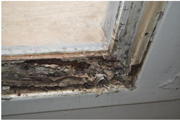
Figure 115. Advanced deterioration and corrosion of the original lower sash and the frame sill (above)
