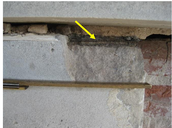
Figure A30. Corrosion scale on strap anchor
