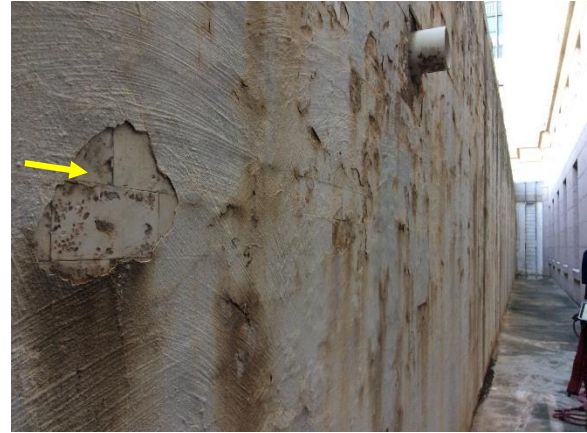
Figure 41. Delaminating tile at light well
