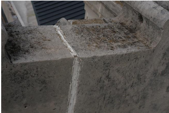
Figure 74. Area of trial cleaning at limestone parapet before application of cleaner
