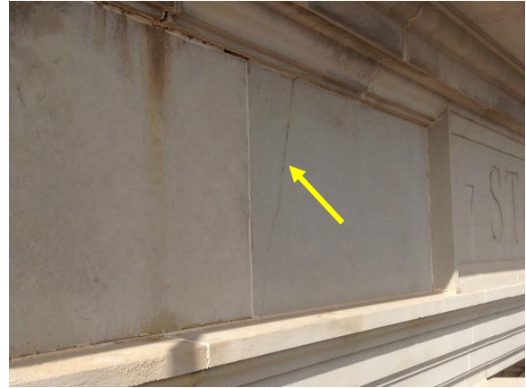
Figure 22. Example of cracked limestone at frieze panel
