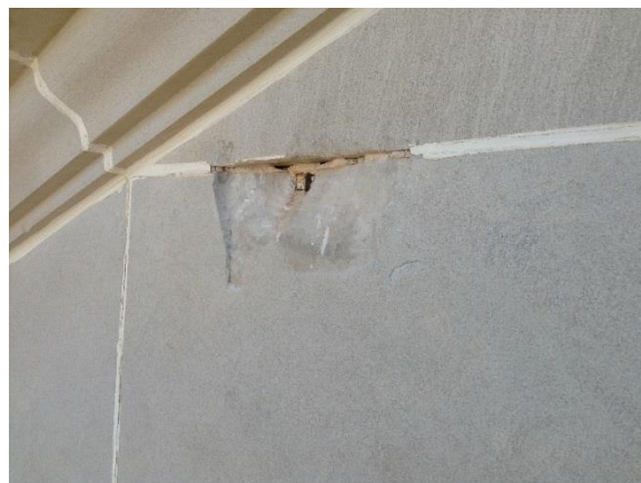
Figure 16. Close-up view of limestone spall at pediment ashlar unit coincident with original strap anchor
