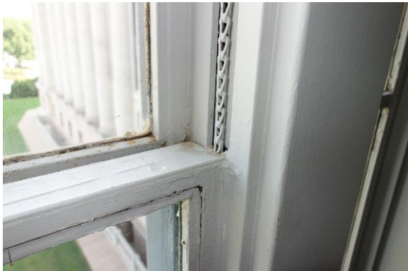
Figure 113. Typical interior condition of the double-hung windows (above)
