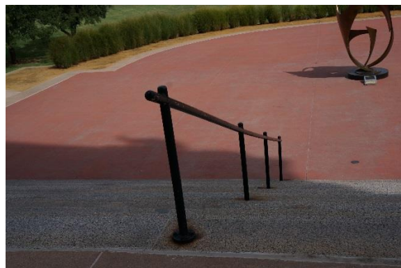
Figure 68. Staining of granite stairs from steel railing
