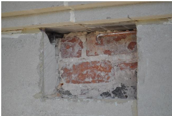
Figure A38. Surface corrosion on cramp anchor
