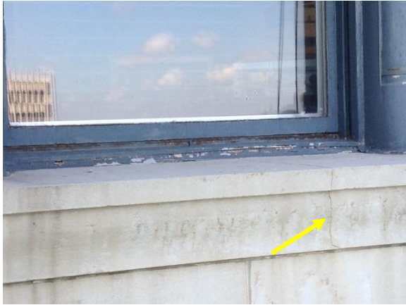
Figure 21. Example of cracked limestone at windowsill
