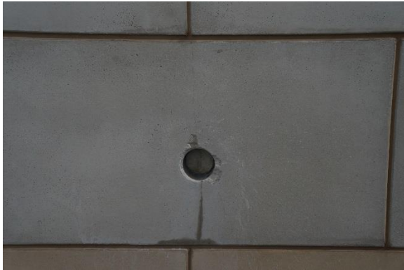
Figure 133. Overall view of core removed from cast stone crack location
