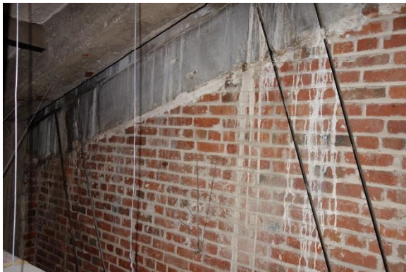
Figure 103. Another view of the metal straps on the west gable wall (above)
