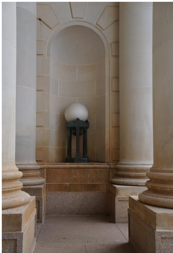
Figure 70. Area of limestone cleaning trials at south portico
