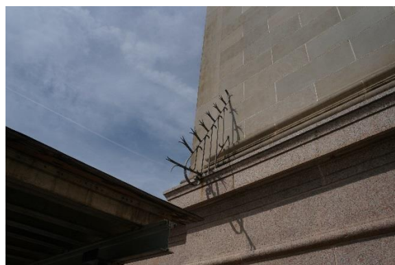
Figure 66. Staining of granite and limestone from surface-applied metal appurtenances
