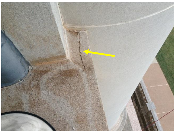
Figure 25. Close-up view of limestone spall at third floor windowsill
