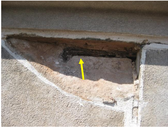
Figure A19. Cramp anchor at crack location
