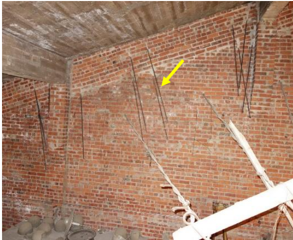
Figure 97. Metal straps that engage two levels of projecting stone work on the exterior of the south gable
