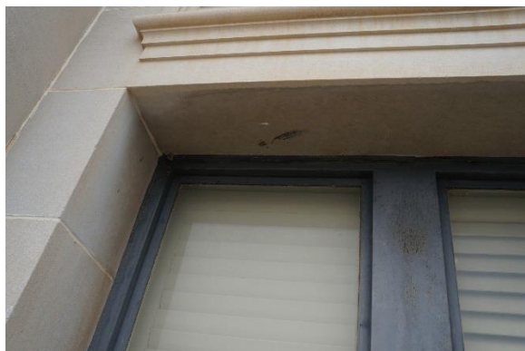
Figure 61. Dark staining below limestone lintels
