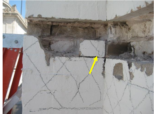
Figure A16. Brick masonry header unit
