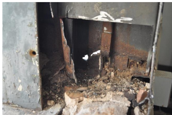
Figure 122. View within the mullion between the two windows
