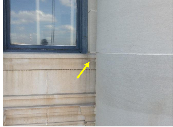
Figure 24. Limestone spall at third floor windowsill
