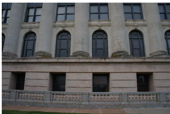
Figure 59. Soiling at limestone column bases above granite
