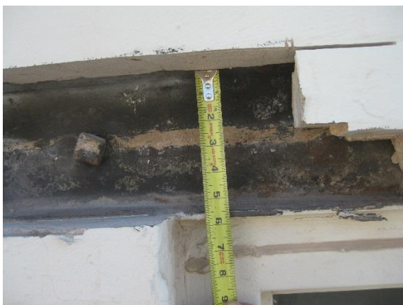
Figure A26. Unengaged bolt at lintel
