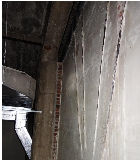
Figure 106. The gypsum panels above the House chamber are cracked.
