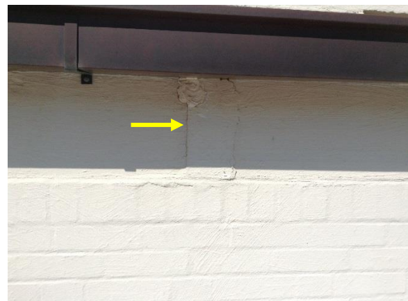
Figure 83. Close-up view of spalling and cracking at back face of parapet wall
