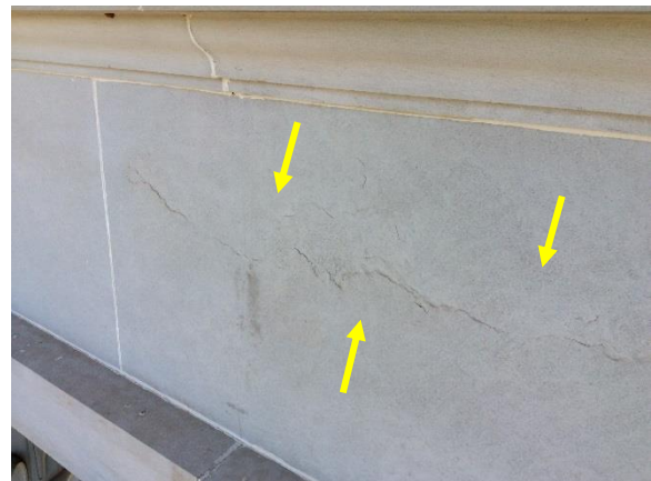
Figure 30. Exfoliation of limestone units
