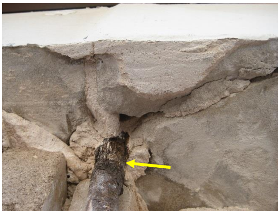
Figure A3. Corrosion scale on anchor rod
