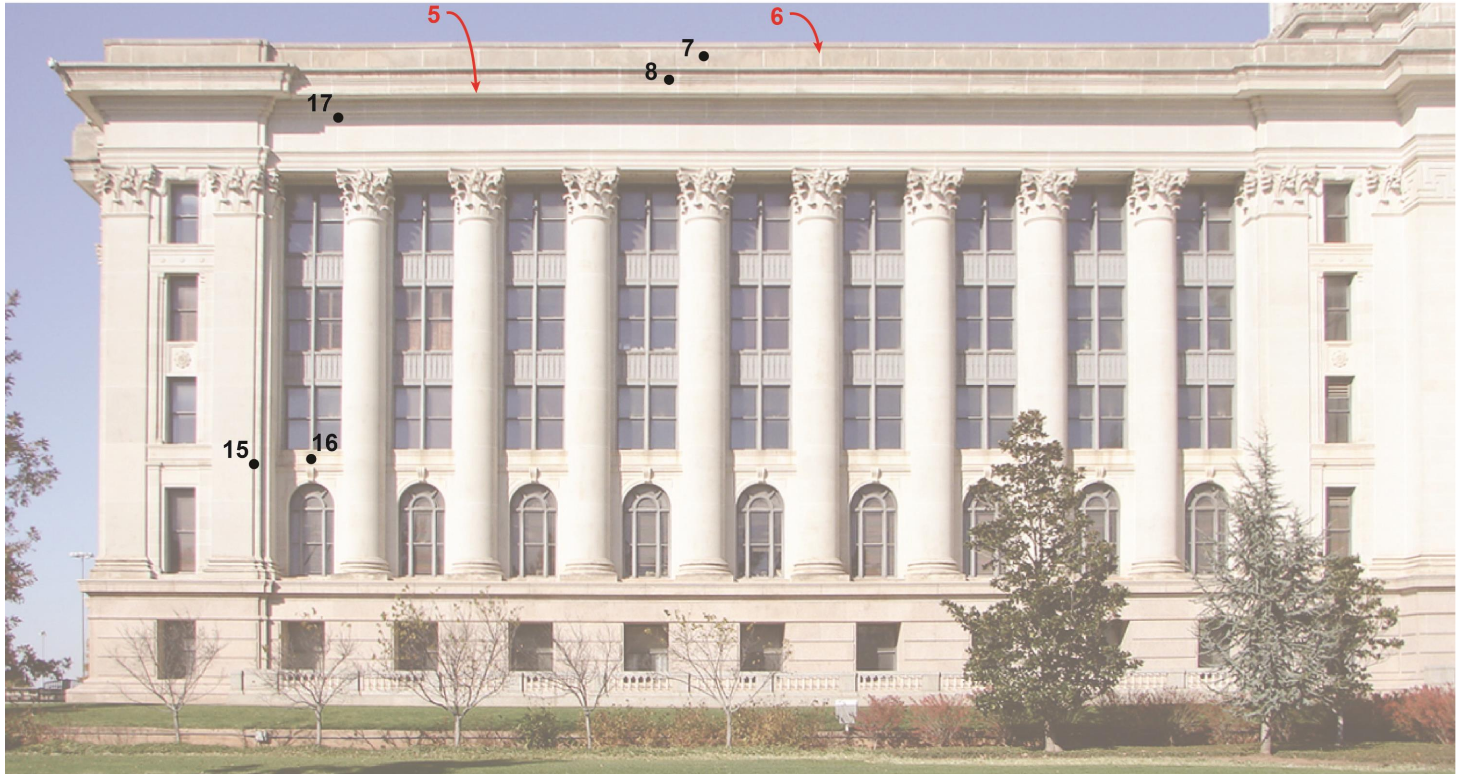
Figure A40. Photograph of south facade, west wing, showing locations of inspection openings. Inspection openings noted in red are on the back face of the facade.
