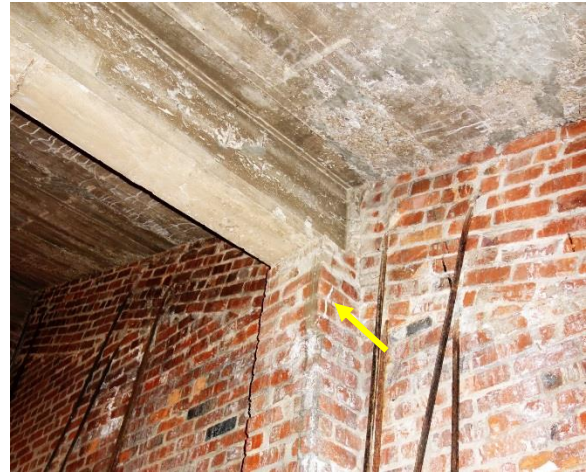
Figure 98. Crack in the corbel at reinforced concrete beam
