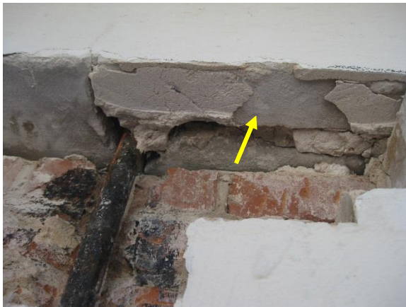
Figure A12. Dutchman unit above inspection opening
