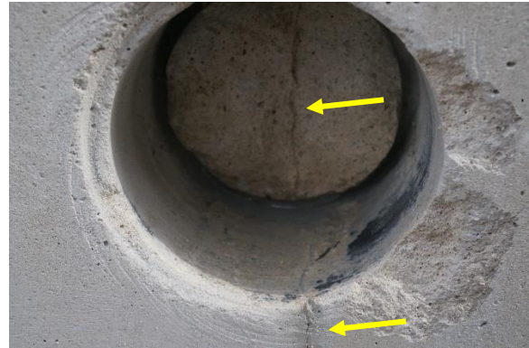
Figure 134. Close-up view of cast stone core removed from cast stone crack location
