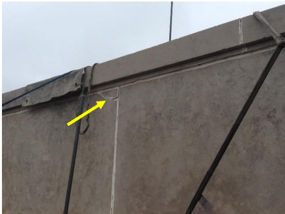
Figure 11. Example of limestone spall observed at parapet wall
