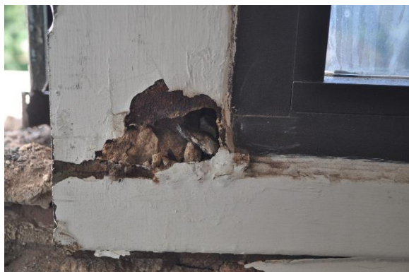
Figure 121. Corrosion of mullion between window sash
