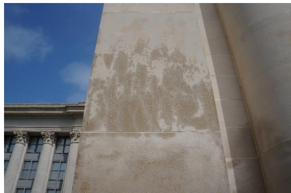
Figure 69. Area of limestone cleaning trial
