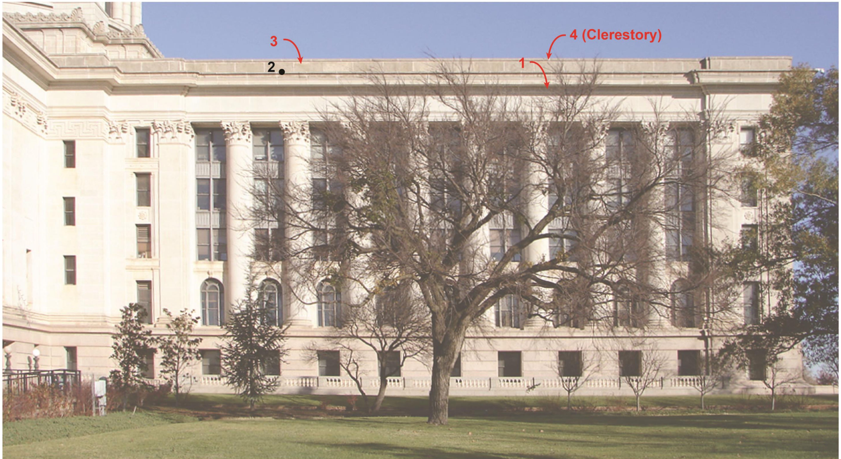
Figure A39. Photograph of south facade, east wing, showing locations of inspection openings. Inspection openings noted in red are on the back face of the facade.
