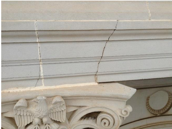
Figure 23. Example of cracked limestone at architrave unit
