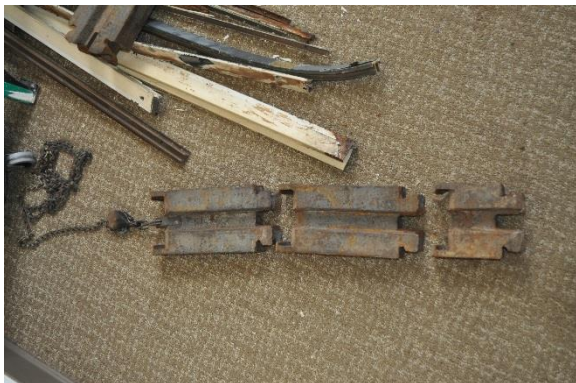
Figure 117. Sash counterweights made of pig iron
