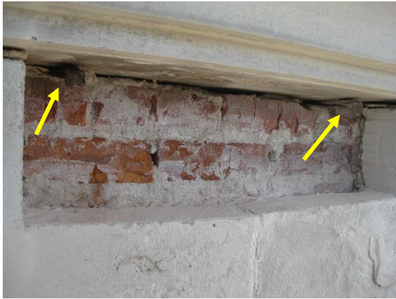
Figure A31. Strap anchors set in brick masonry backup
