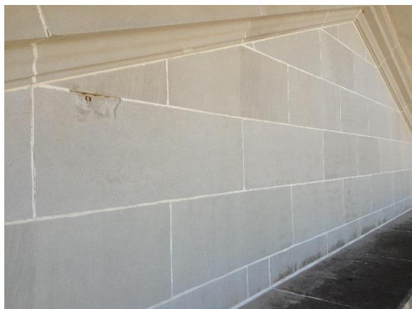
Figure 15. Example of limestone spall at pediment ashlar units
