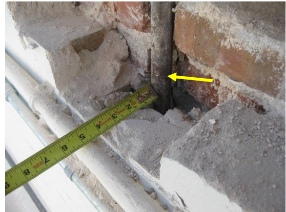
Figure A2. Cornice anchor rod
