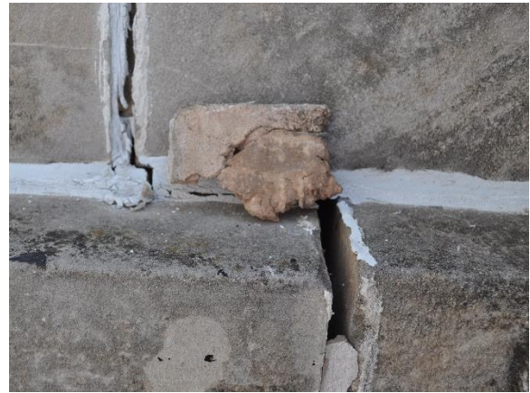
Figure 28. Washed-out mortar joint
