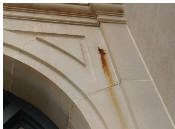
Figure 32. Mineral inclusion in limestone causing iron oxide staining
