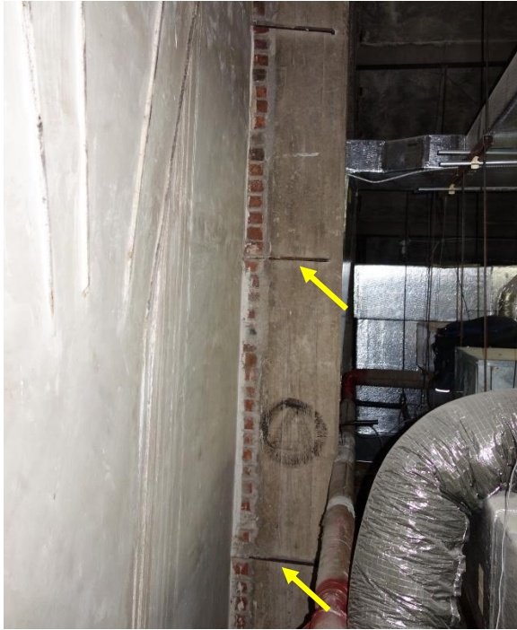
Figure 109. Metal anchors that connect the masonry of the east gable to the concrete frame
