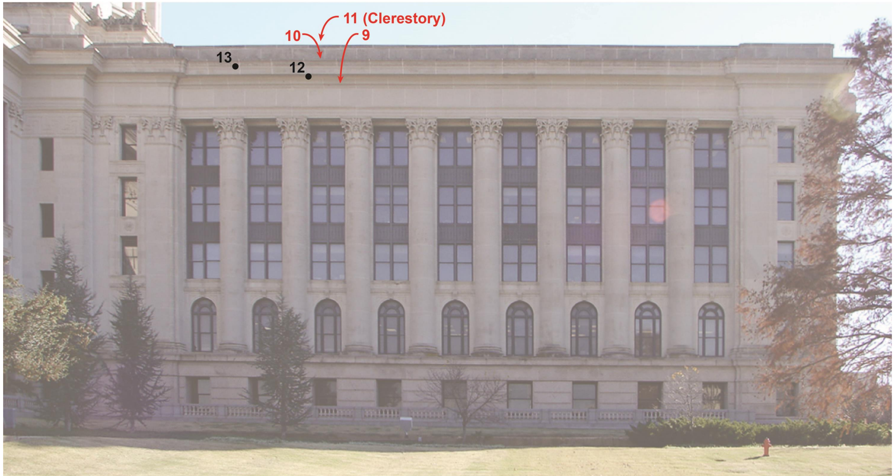
Figure A41. Photograph of north facade, east wing, showing locations of inspection openings. Inspection openings noted in red are on the back face of the facade.
