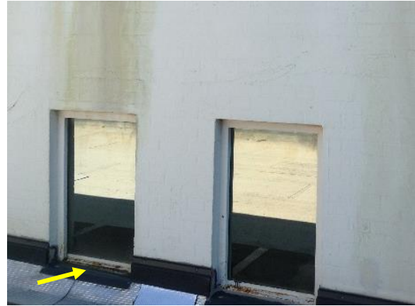
Figure 89. Corrosion staining at clerestory windowsill
