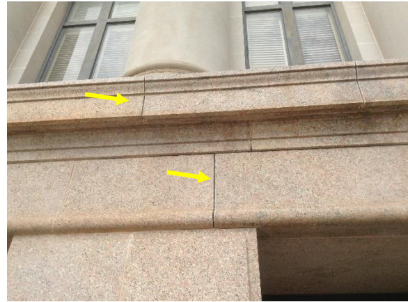
Figure 39. Washed-out mortar in granite units
