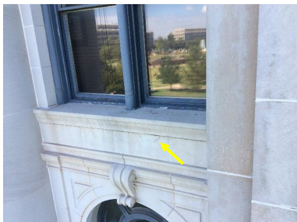
Figure 17. Example of limestone spall at spandrel panel
