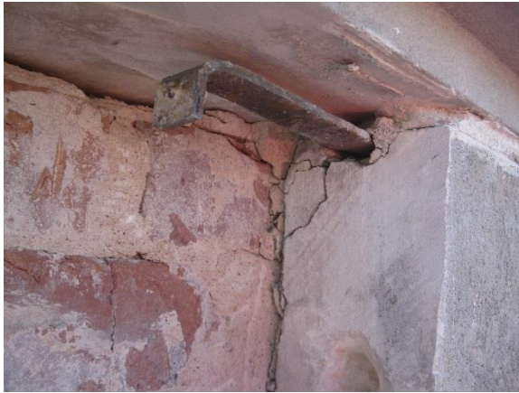
Figure A27. Cramp anchor between limestone panels
