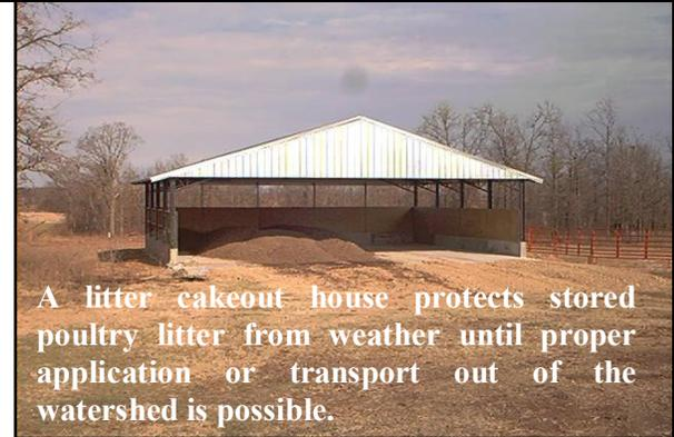
A litter cakeout house protects stored poultry litter from weather until proper application or transport out of the watershed is possible.
